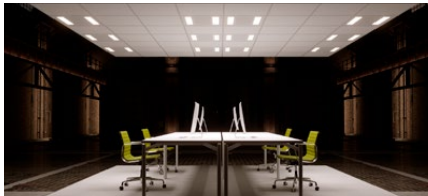
After, with Linessa Air and integrated ventilation.
